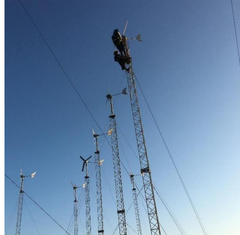
Figure 16. Process of installing blades on the pole
